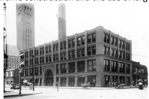
The building shown is only four stories tall. Seven more floors were added in 1909. Note the early car at left and the man with the vegetable cart. Hennepin County Library
